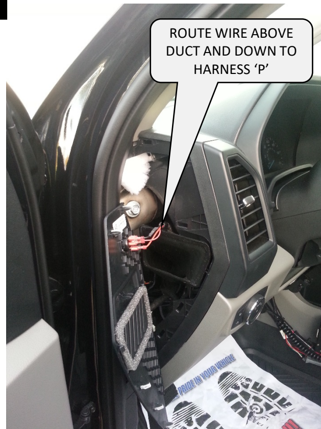
AFTER REMOVAL OF FACTORY TRIM PANEL, REPLACE WITH TRIM PANEL WITH SWITCH. RUN HARNESS 'O' DOWN TOWARD HARNESS 'P' CONNECTOR
