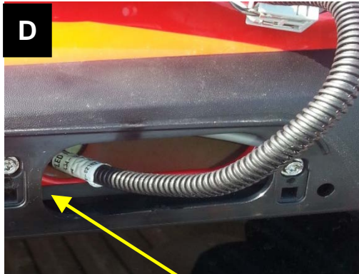
D FEED CHMSL HARNESS THROUGH BEZEL & DOWN INTO CABIN ACCESS HOLE.
